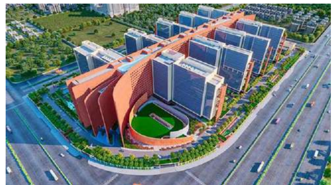
Surat diamond bourse Aerial view
